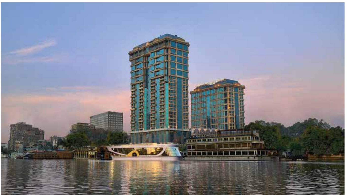
Four Seasons Hotel, Cairo -Trust provided Ecology systems for commerical kitchen
